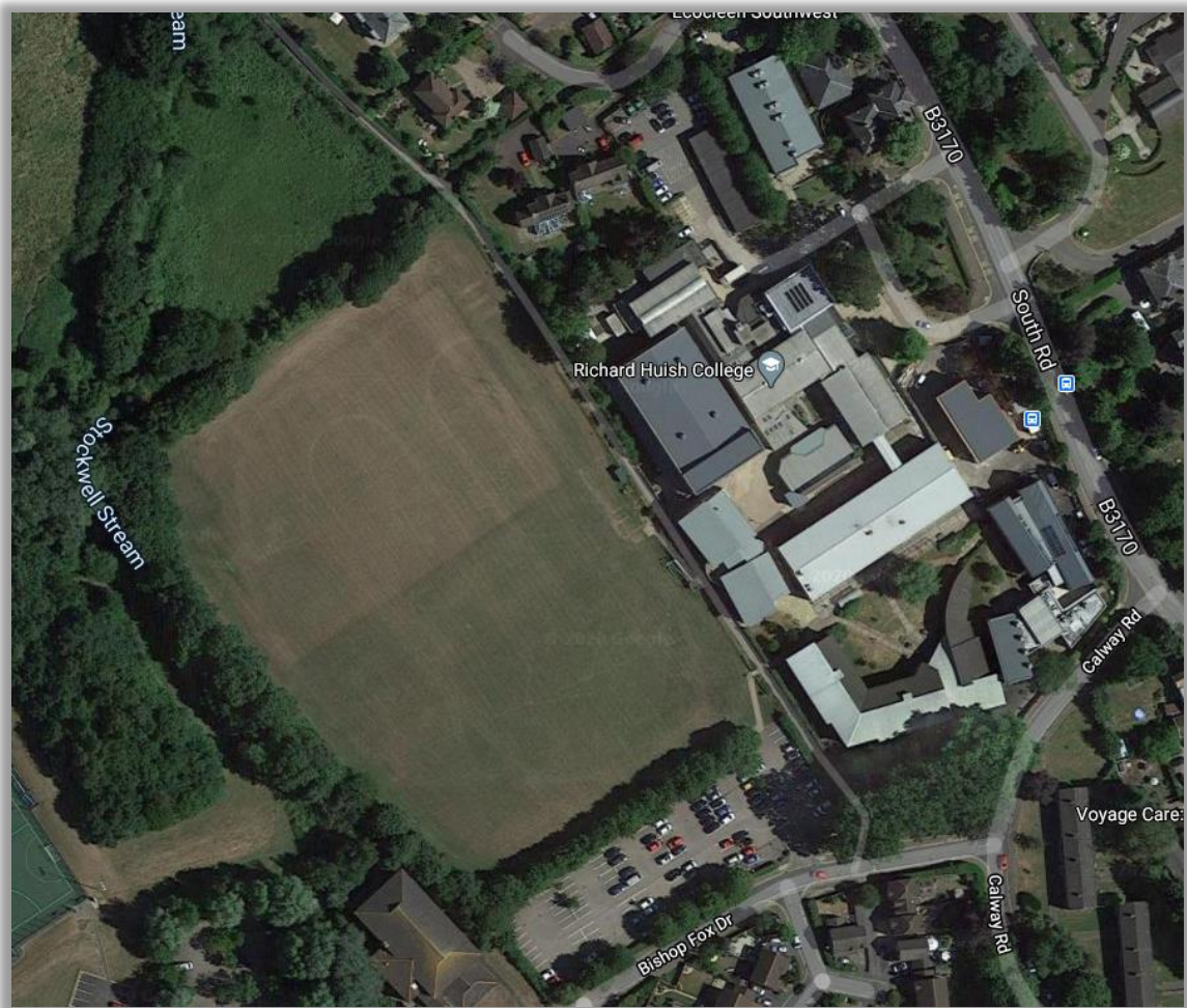
Figure 13: College site (aerial)
