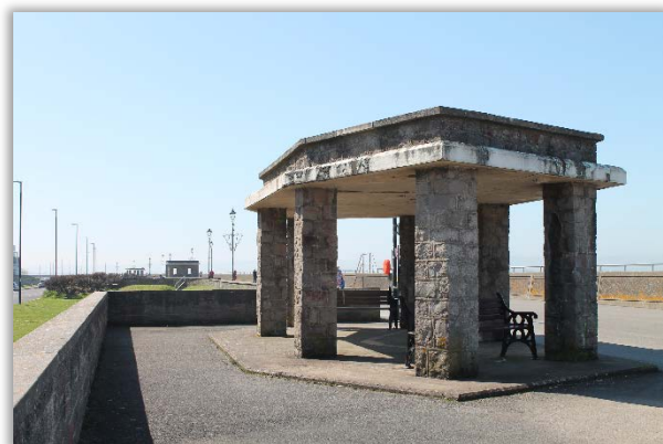
Shelters on South Esplanade need replacing
