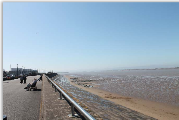
Extensive functional (yet) bland sea wall
