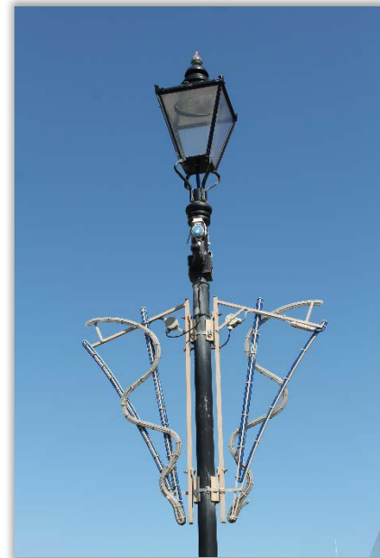
Poor quality lighting on South Esplanade
